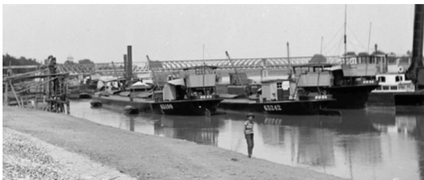
Railway bridge of Osijek over the Drava in 1922. In the foreground DDSG barges. (Fortepan 2784)
